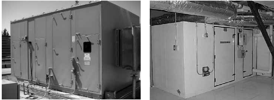
Figure 4.01 Interior and Exterior Air Handling Units
